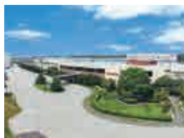
CHINA China Plant (MCC)
